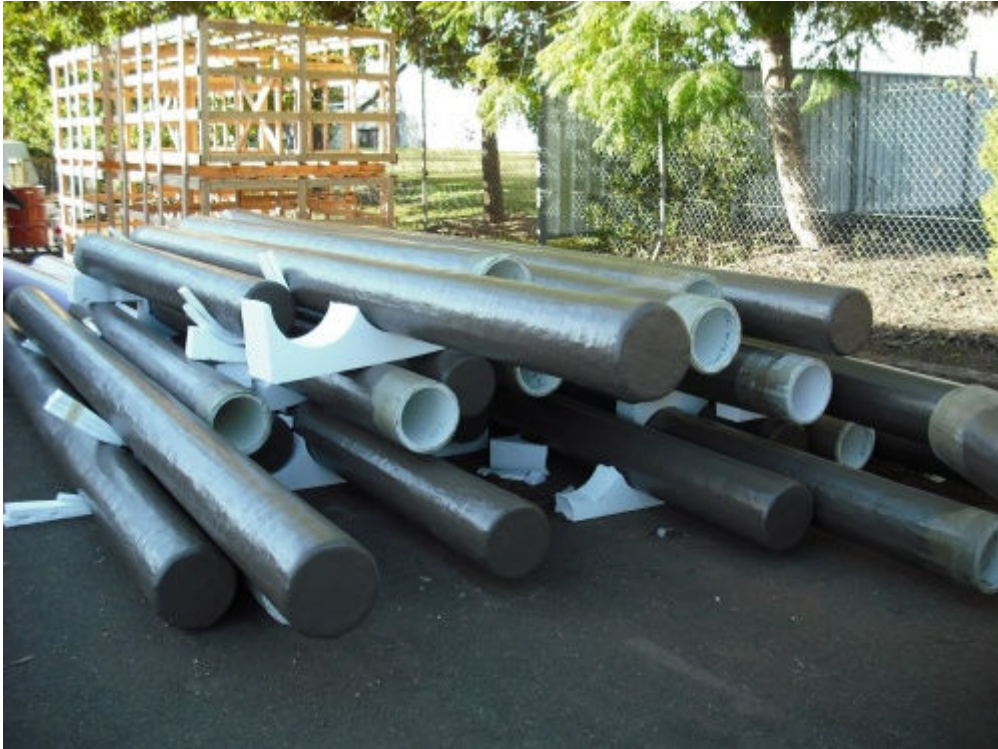
BAC piles for Shorncliffe Pier
